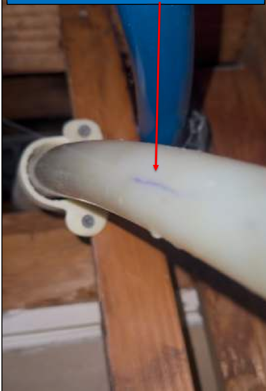
Image 7- Representative cracked and leaking Uponor PEX white pipe away from fitting
